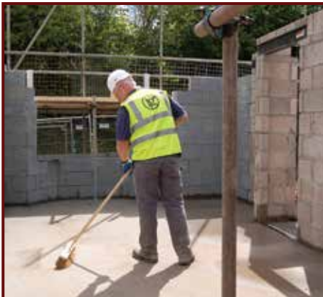
1. Clear debris from work area
