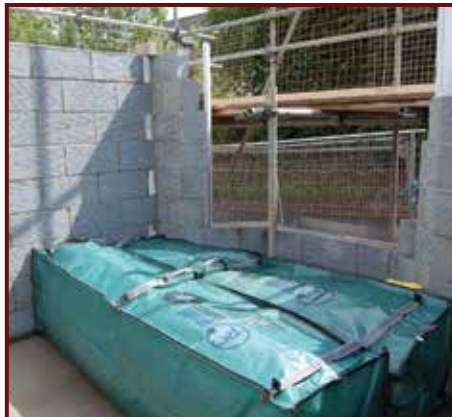
2. Load bags into work area and place in position
