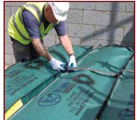
3. Check clips are free of debris
